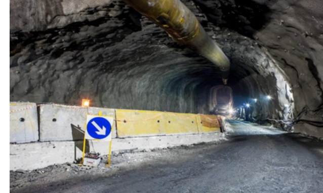
Jurong Island Tunnel in Singapore
