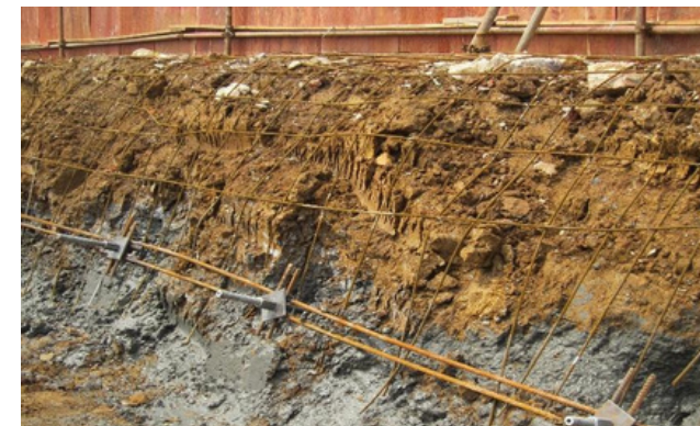
Nanjing Zijin investment side slope support
