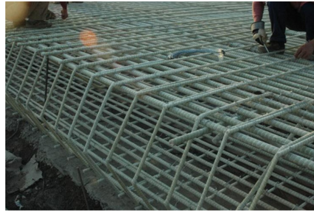
Cross-river tunnel underground continuous wall project
