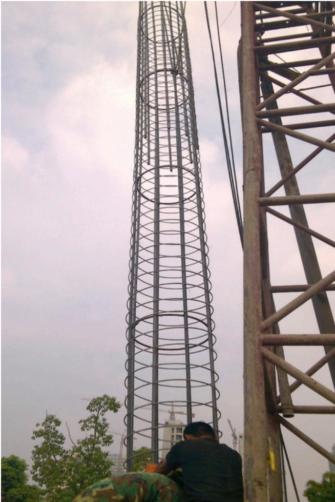
Jiangsu Provincial Food and Drug Administration Foundation Pit Project
