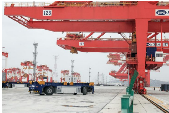
Shanghai Yangshan Port Automation Wharf Project
