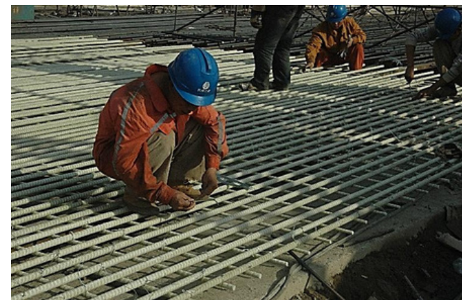
Subway Connecting Wall Project
